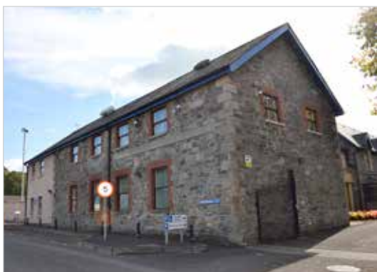
Strabane District Council buildings
