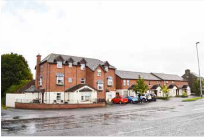
Public Authority Housing at Mill Place, Limavady
