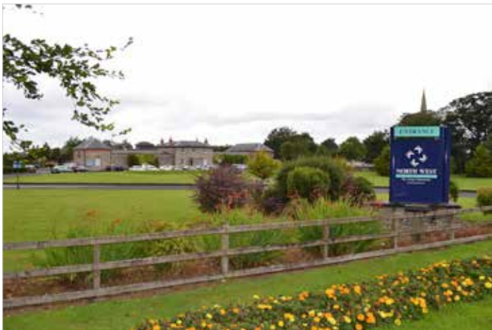
Northwest Independent Hospital, Ballykelly
