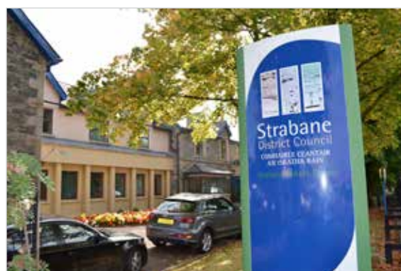
Strabane District Council buildings
